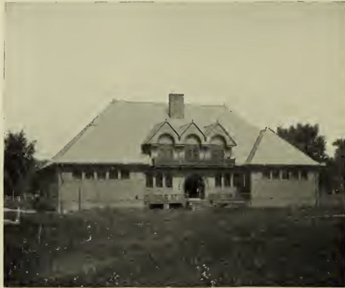
CAREY BUILDING, HOLMES FIELD
